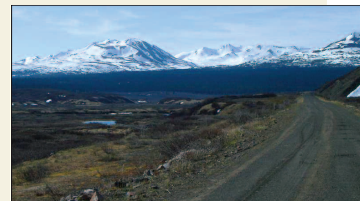
Railway sub-grade links mine site with CN mainline & Ridley Terminals
